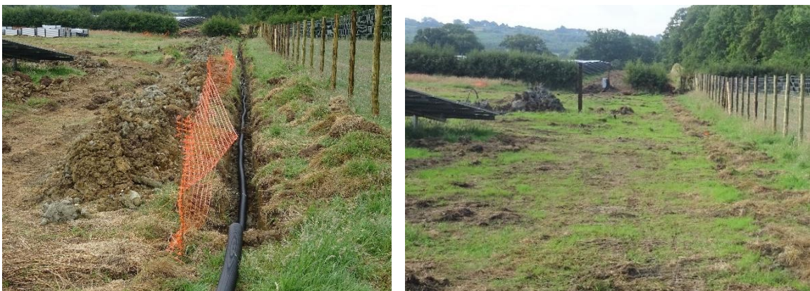
Figure 15.15-16 Cabling Channels during Cable Installation
