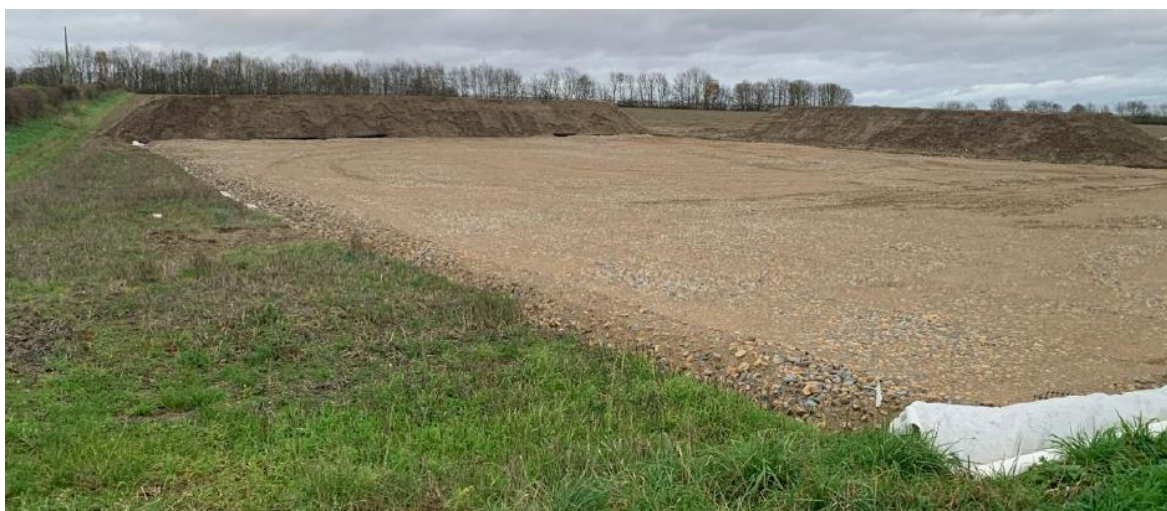
Figure 15.14 5 Newly Installed Construction Compound
