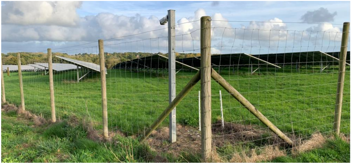
Figure 15.17-18 Typical Deer Fencing
