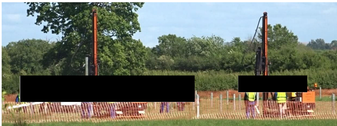
Figure 15.10-11 Mounting Structure Piles being Installed
