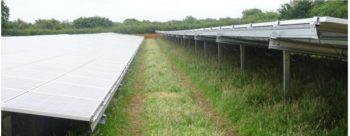
Figure 15.12-13 Part Installed Panels (Bentham Farm, Purton)
