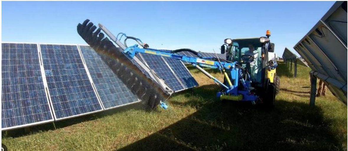
Figure 15.19-20 Cleaning of Solar Modules
